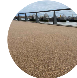
RESIN BONDED GRAVEL Yellow colour, slip resistance
